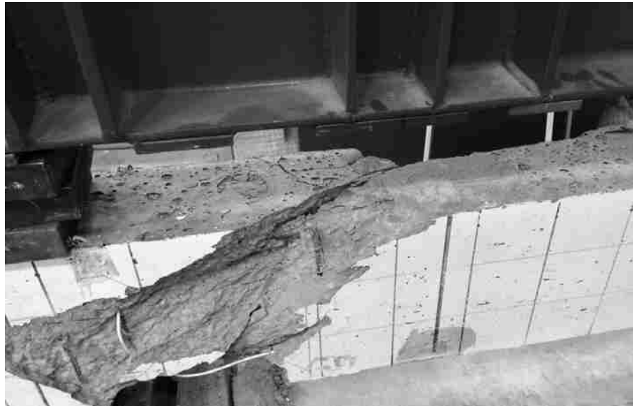
Fig. 12. Failure mode of GL6-2
